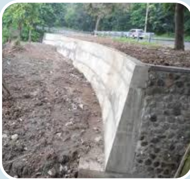
Bored Pile Foundation to Protect slope
